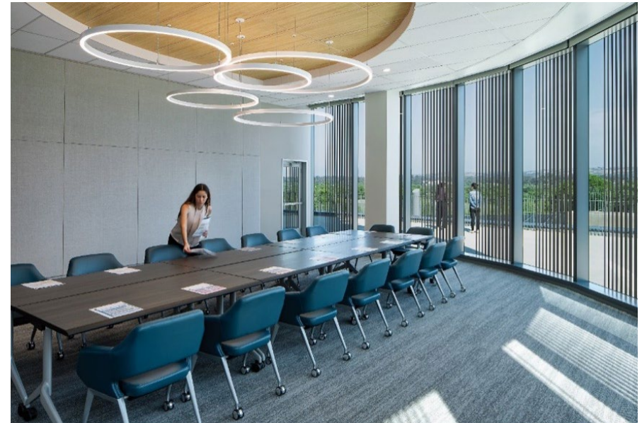
The unitized curtainwall combines full-height glazing for views of the marsh with Fibonacci sequence frits that progressively double in thickness. Functionally, the frits control heat gain and discourage bird strikes. (Tom Bonner/Courtesy CO Architects)
